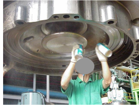
Combustion chamber after cleaning.
